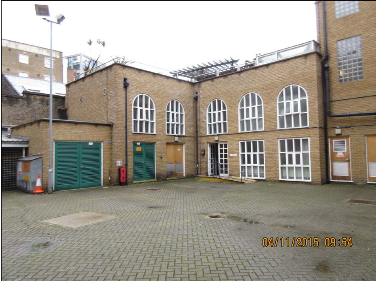
Existing buildings at the rear of the fire station
